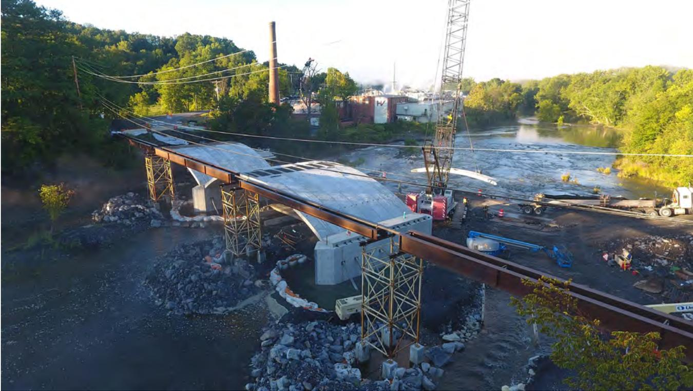
*Construction – During the Erection of the New Bridge*
